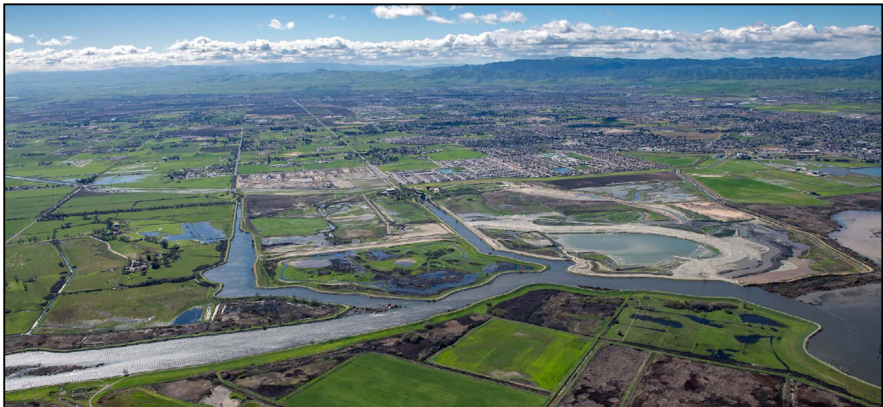
A view looking south of the Dutch Slough Tidal Marsh Restoration Project in the Sacramento-San Joaquin Delta near Oakley, Calif. Photo by Ken James, Department of Water Resources.
