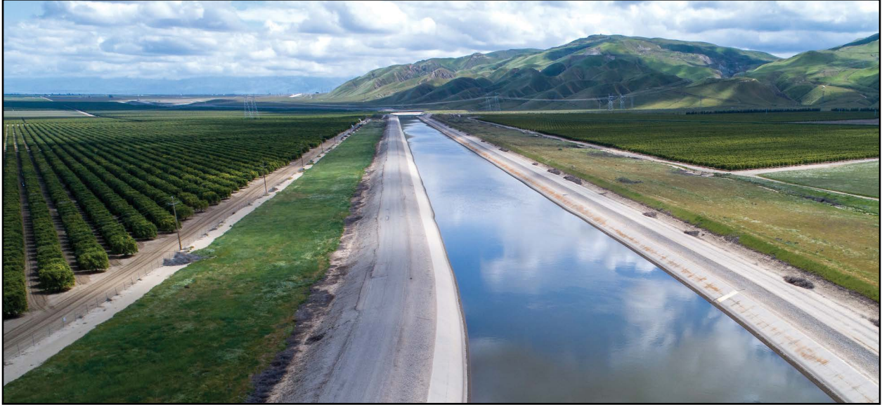
A section of the California Aqueduct within the State Water Project in Kern County. Photo by Ken James, Department of Water Resources.
