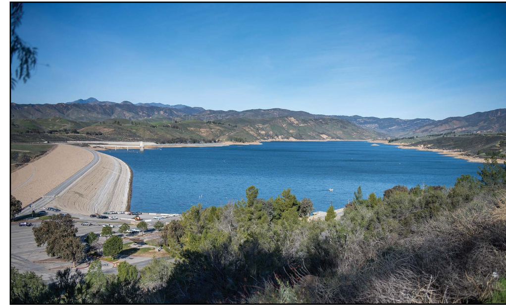
Castaic Lake is a reservoir formed by Castaic Dam on Castaic Creek, in the Sierra Pelona Mountains of northwestern Los Angeles County, California. In 2018, DWR completed spillway inspections, assessments and maintenance efforts on seven SWP dams: Pyramid, Castaic, Cedar Springs, Grizzly Valley, Frenchman, Antelope, and Del Valle. Source: Department of Water Resources
