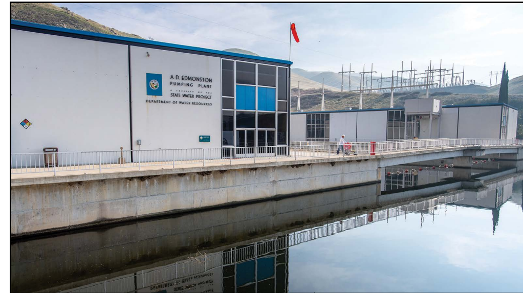
Located at the base of the Tehachapi Mountains in Kern County, the A.D. Edmonston Pumping Plant provides the largest lift within the California Department of Water Resources State Water Project system. Source: Department of Water Resources
