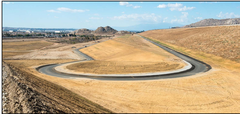
The seismic remediation of the dam embankment has been completed at Lake Perris in Perris, California. Perris is located in Riverside County. Photo taken February 23, 2018. Source: Department of Water Resources
