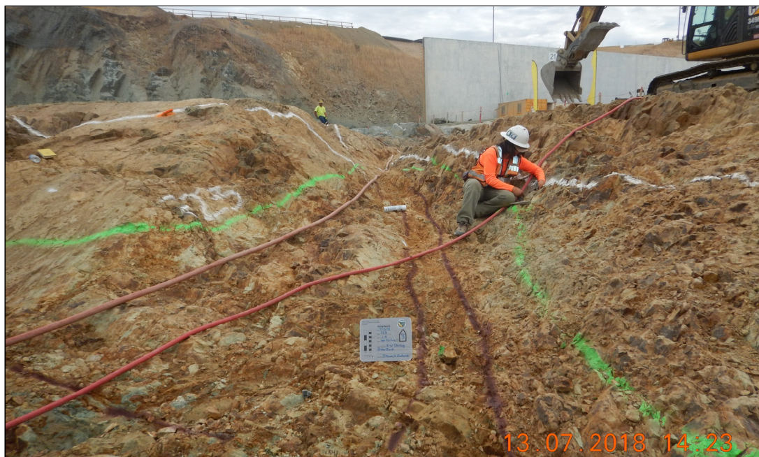
Figure 4. Example of local more highly-weathered zone (between green paint lines) in FCO bedrock foundation.
