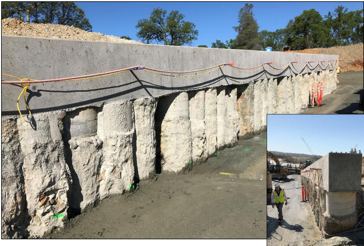
Figure 1. Photographs Showing RCC Apron (Top) and Secant Pile Wall (Bottom)
