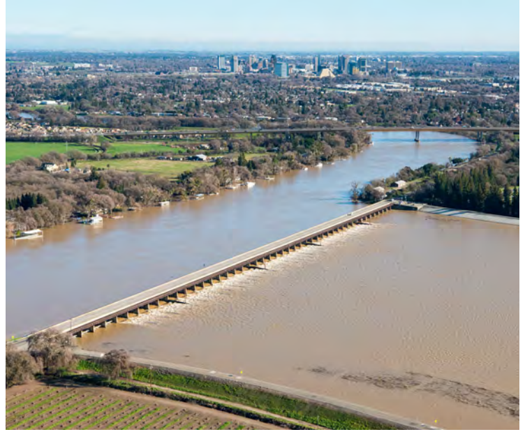
Gates on the Sacramento Weir were opened in 2017 to allow water to flow from the Sacramento River into the Yolo Bypass. The 1,920-foot long weir, constructed in 1916, is one of multiple structures making up the Sacramento River Flood Control Project. Its manually operated gates are opened based on forecasted river flows to reduce Sacramento River flood stages downstream of the American River confluence, to reduce flood risk to the metropolitan Sacramento area. Prior to water year 2017, the gates were last opened in December 2005.
