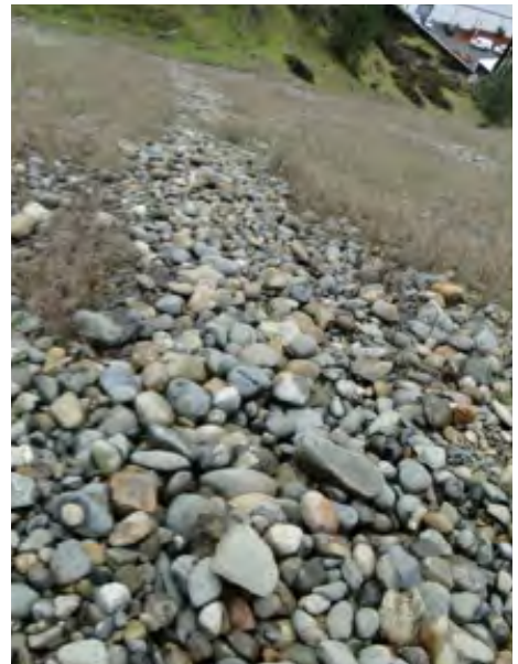
FIGURE 16. Eroded rills or gullies in the vegetation area that were filled with cobbles. This encourages rain water percolation into the fill instead of running down the slope. (Photographs taken January 20, 2017)
