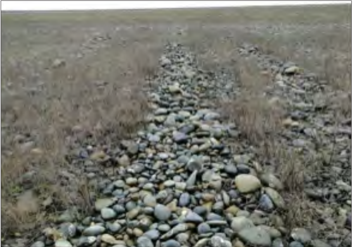
FIGURE 16. Eroded rills or gullies in the vegetation area that were filled with cobbles. This encourages rain water percolation into the fill instead of running down the slope. (Photographs taken January 20, 2017)
