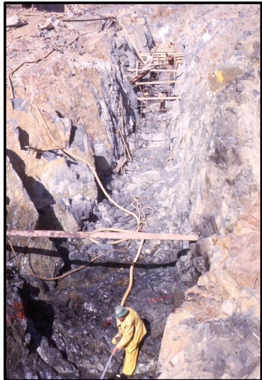
Figure 3: Photographs of Slightly Weathered Rock Exposed in Excavation of Grout Gallery on Right Abutment of Oroville Dam (from DWR Photography Files)
