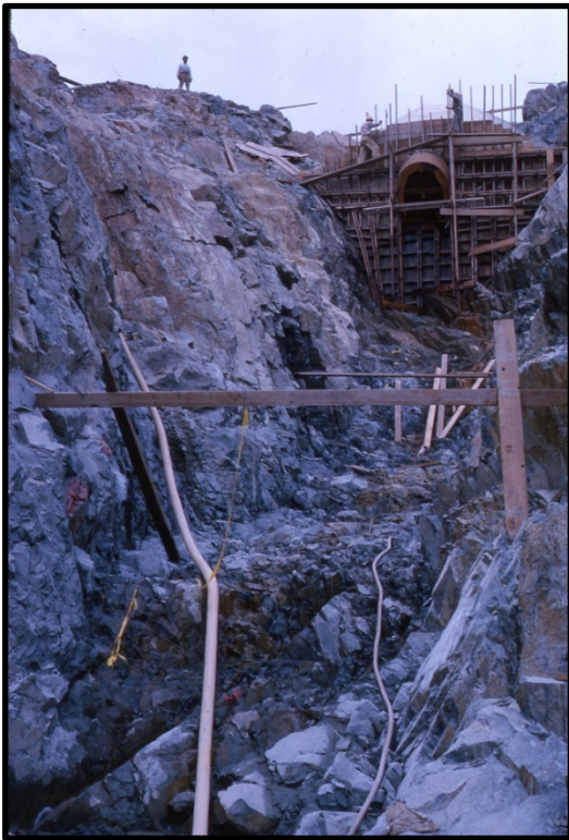
Figure 3: Photographs of Slightly Weathered Rock Exposed in Excavation of Grout Gallery on Right Abutment of Oroville Dam (from DWR Photography Files)
