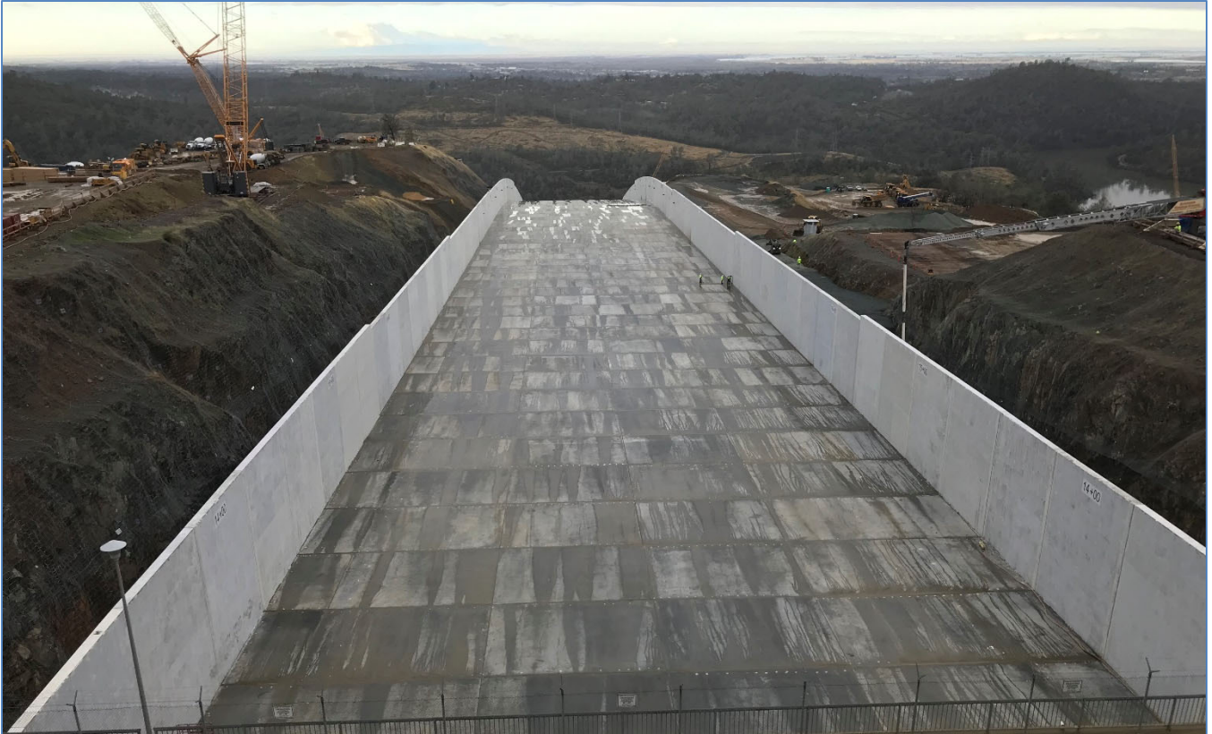
Figure 1. Completed FCO Chute.
