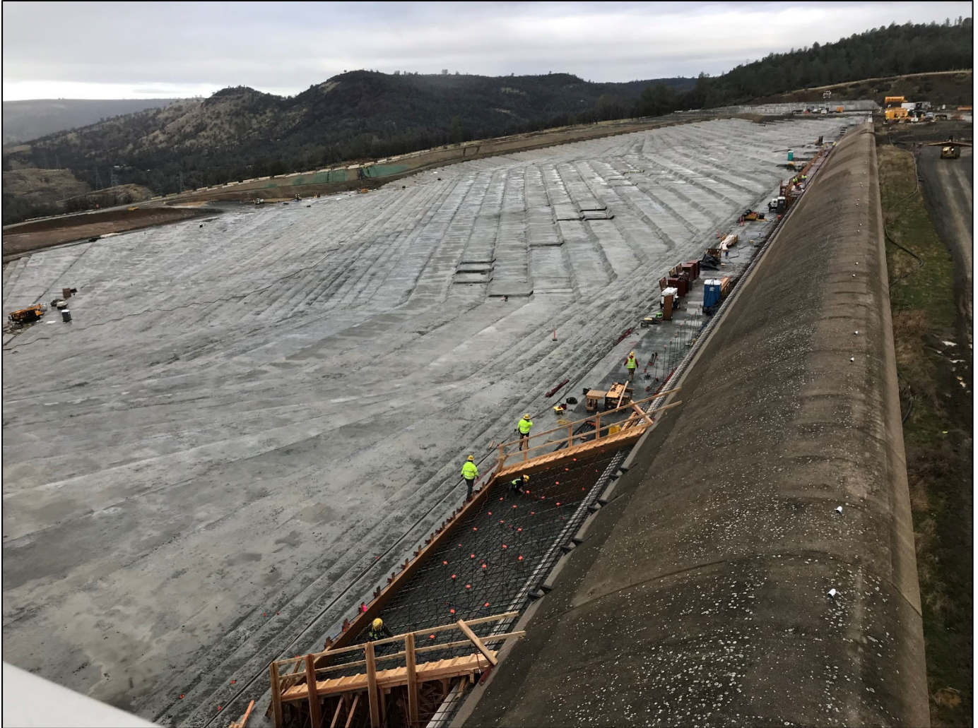
Figure 3. Emergency Spillway RCC Apron and Buttress formwork.
