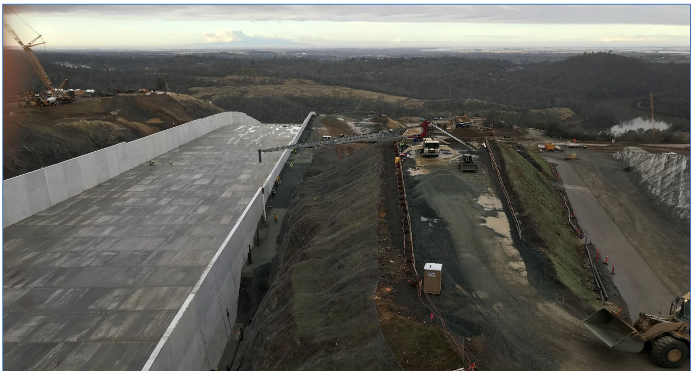
Figure 2. Placement of backfill behind FCO chute walls.
