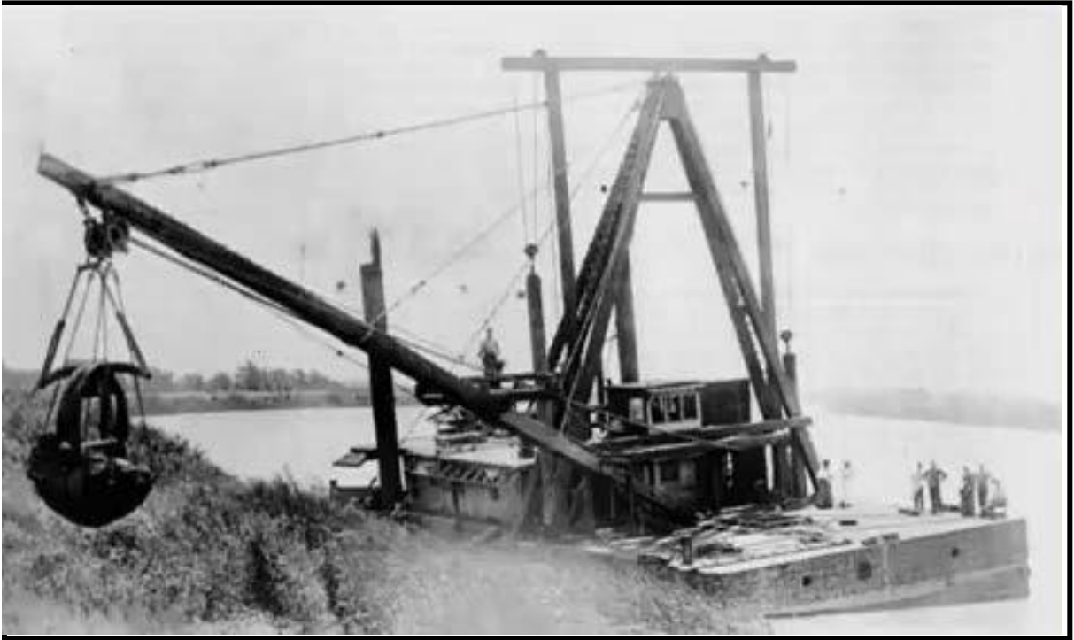
Figure 3-3. Clamshell Dredge. Image courtesy of Maven’s Notebook, 2017.
