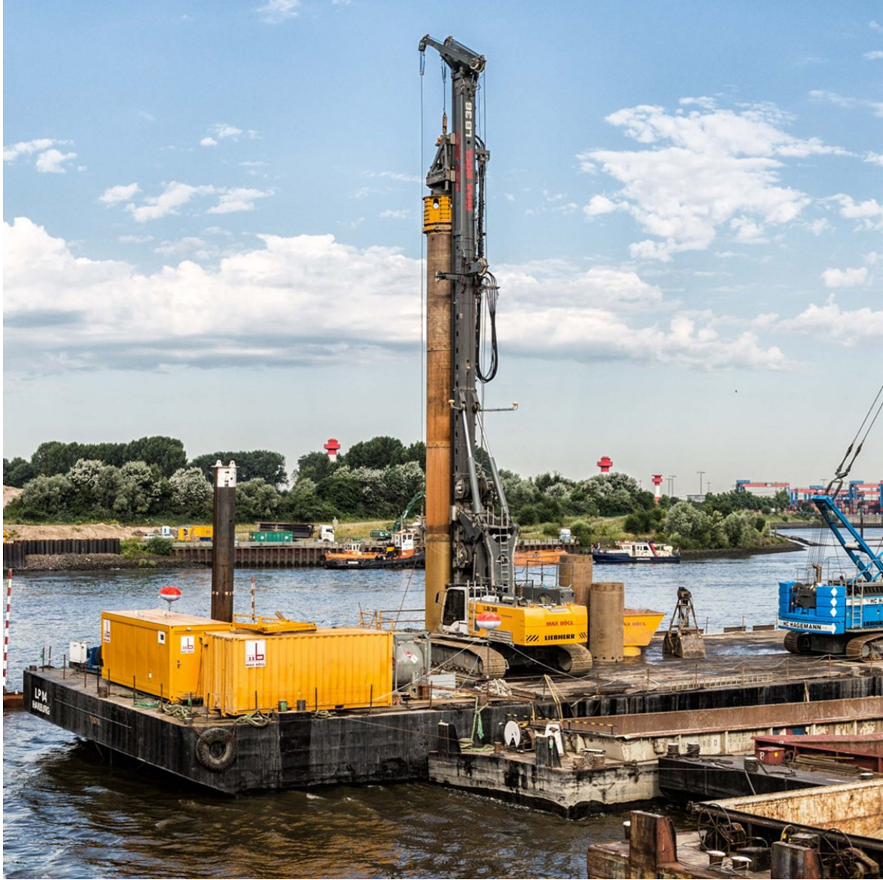
Figure 11. Barge-mounted Rotary Drill Rig
