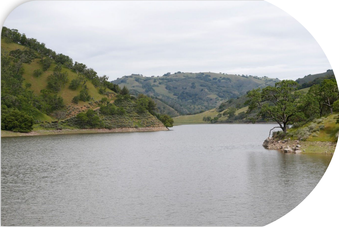
Pictured above: Existing Pacheco Reservoir
