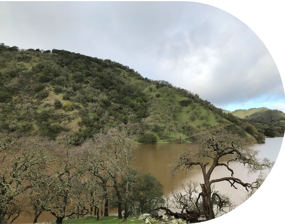
Pictured above: Existing Pacheco Reservoir
