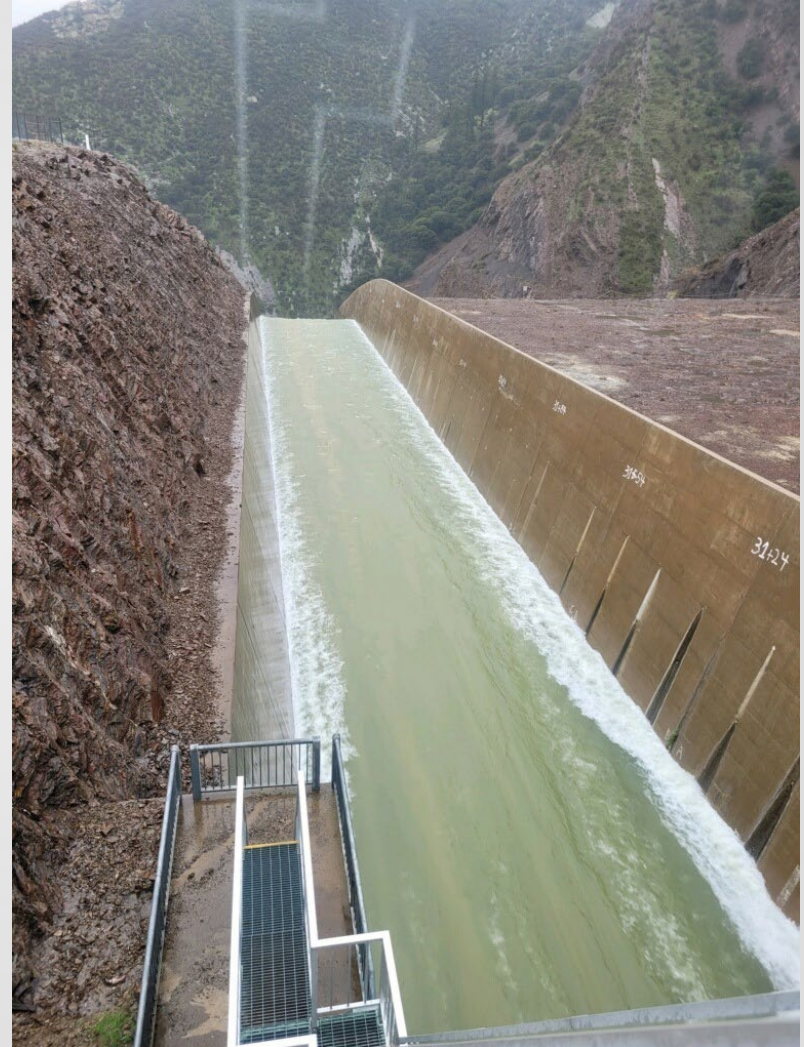
Pyramid Dam's Spillway
