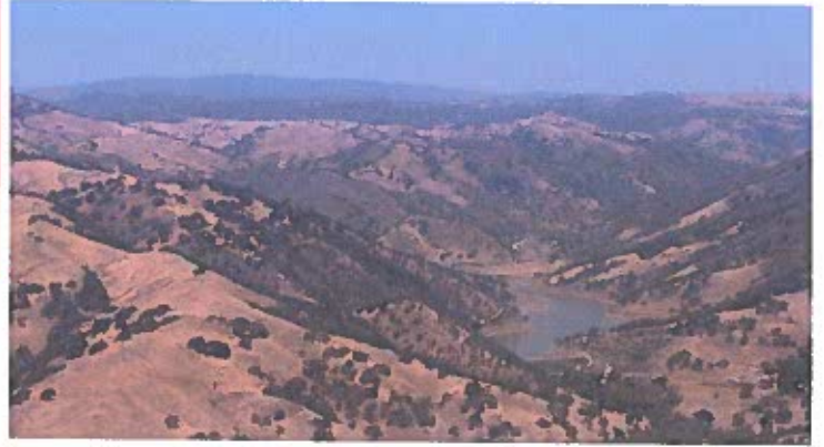
Aerial view of Pacheco Reservoir
