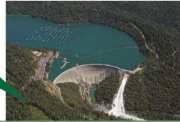
▲ New Bullards Bar Dam
