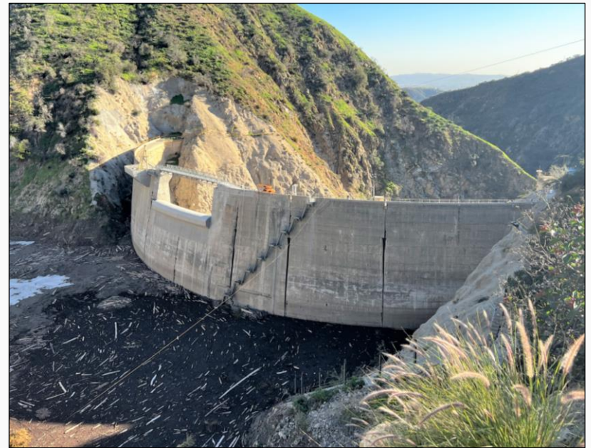
January 2023 Sediment level El. 1,246 ft.
